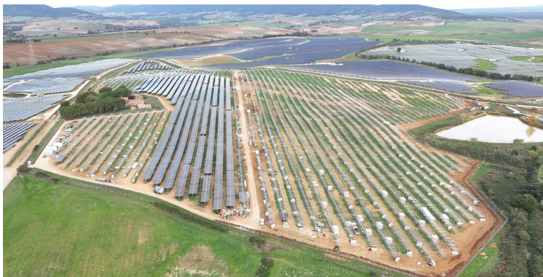
CCEs PV-plant in Montalto di Castro, Italy. ©CCE
